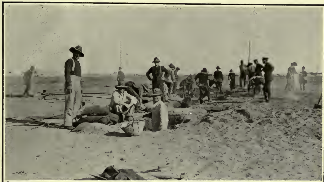
TRENCH DIGGING IN THE DESERT SANDS. Party of the New Zealand Contingent in Egypt.
