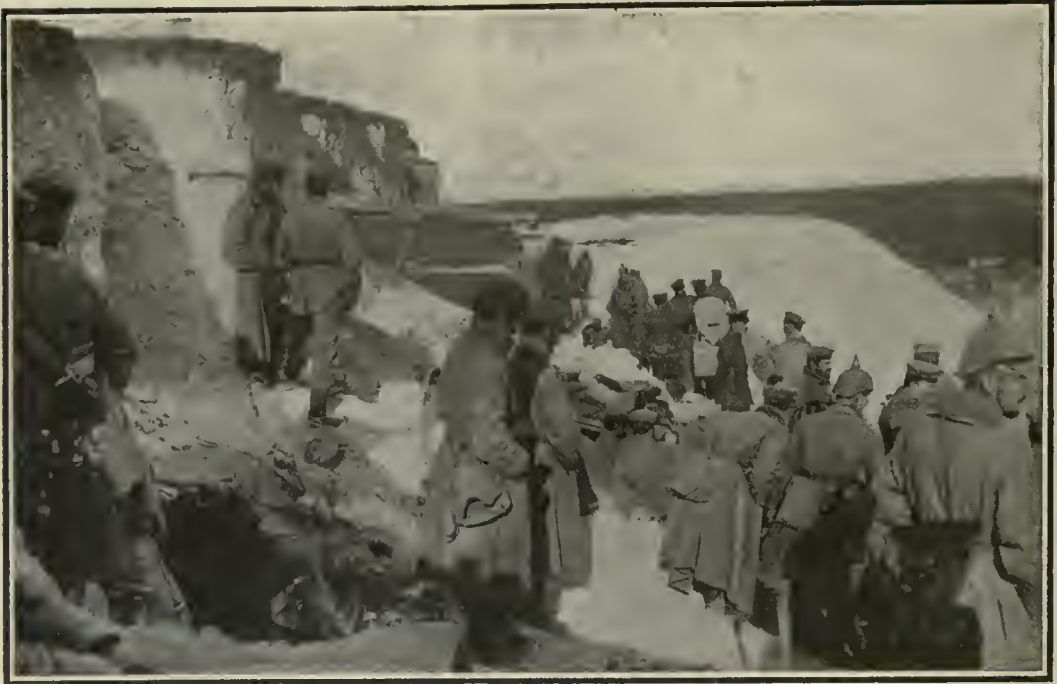
NORTH-WEST OF HULLUCH. The Quarries occupied by the Germans.
