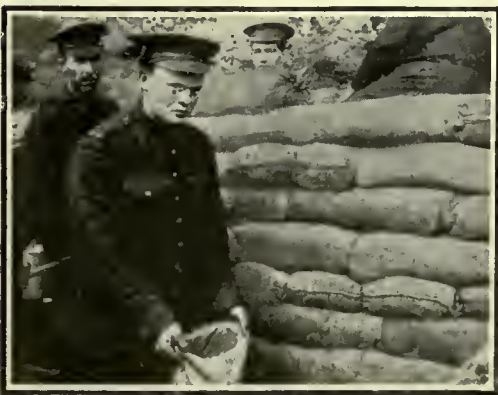
BUILDING A TRAVERSE IN A FRONT-LINE TRENCH.
