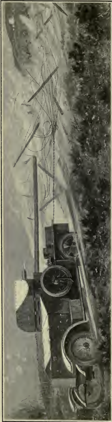
AN ARMoured CAR OF THE NAVAL DIVISION "GRAPNELLING" WIRE ENTANGLEMENTS. A British car in Gallipoli uprooting and tearing down barbed-wire defences in front of a Turkish trench.
