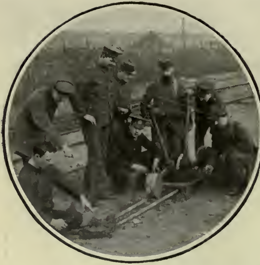
Repairing a railway point.
