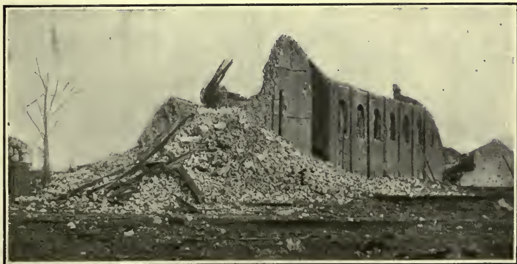
AFTER THE BRITISH ATTACK. A wrecked church in Loos.
